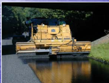
Rubberized Asphalt Chip Seal
