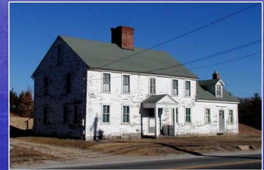
Reuben Mason House Restoration – Glocester
