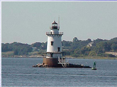
Conimicut Shoals Lighthouse Restoration – Warwick
