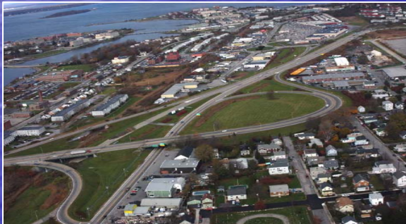
Pell Bridge Ramps
