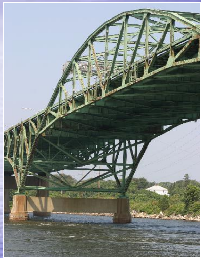
Sakonnet River Bridge
