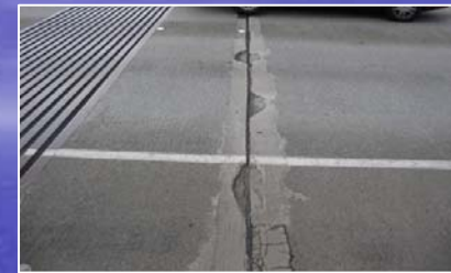
Deck Joint Repair
